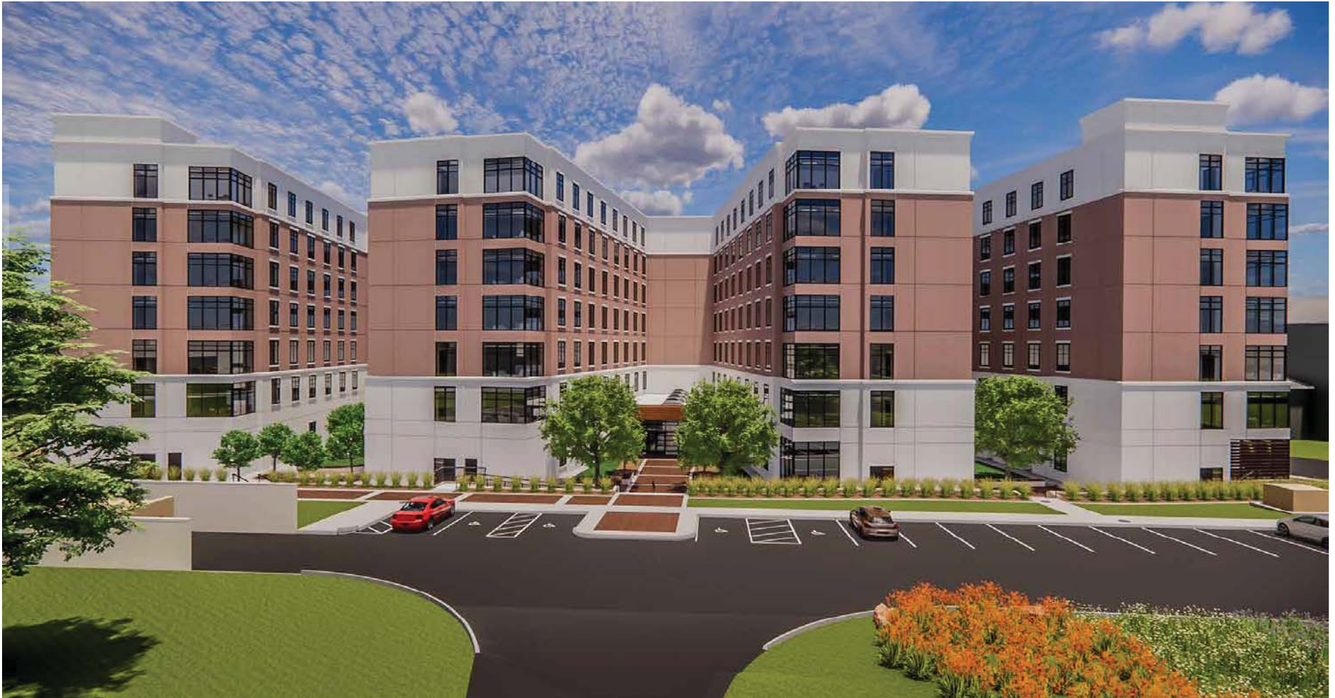
View from North - Main Entrance
